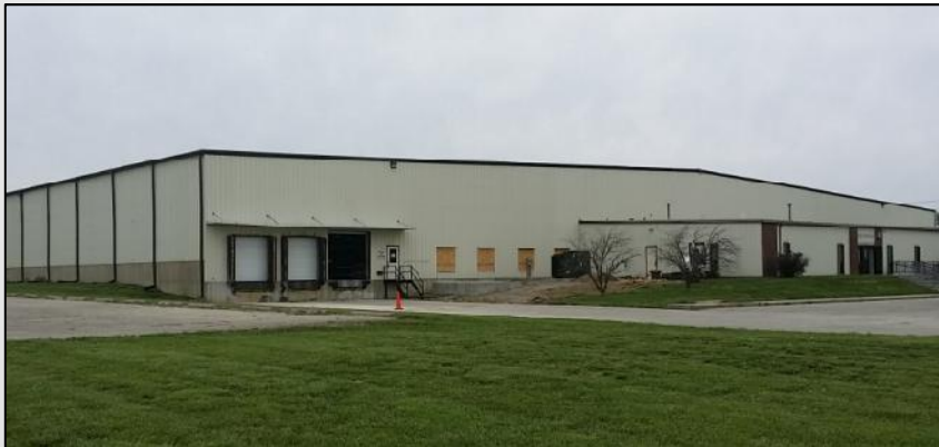
Warrensburg, Missouri Facility
